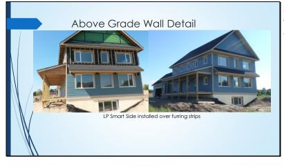
Siding installation over the furring strips after the insulation was completed
