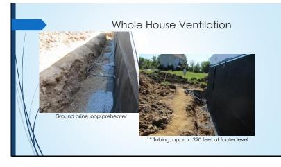
The optional geothermal loop will help temper in the cold winter air before it goes to the air to air heat exchanger and will provide dehumidification in the summer. We can get roughly a half ton of cooling for the electrical load of about 25 watts. - around 240 SEER
