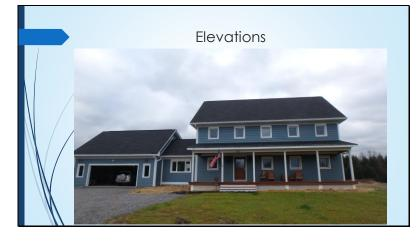
Front of the house faces due west. Smaller windows, lots of shading where possible to help control the solar gain from the west. We also had the windows glazed for a SHGC for 0.3 on the west side of the house.
