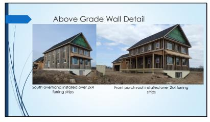
Now we added the overhangs and front porch roof. We have a complete thermal break between the roofs and the structure of the house. With all of this installed we insulated the wall assembly with dense packed cellulose.
