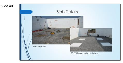
Prepped for slab pour with crushed stone, added 8" of EPS foam under post location. The EPS foam used has a compressive strength of 40 PSI (5760 PSF) – Assumed soil bearing pressure is 3000 PSF.
