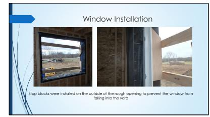
Now we installed shims on the bottom where necessary. Installed our stop blocks and set the windows in place
