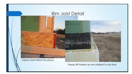
1<sup>st</sup> floor AGW built and floppy bit flopped up over rim board.
