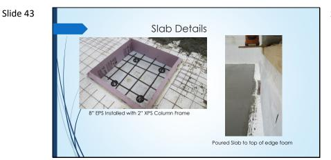
Slab edge insulated with 8" of EPS foam plus R-20 ICF.
