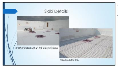
8" EPS foam laid down sub slab. Post column frame made out of foam. This will help minimize "floating the foam".
