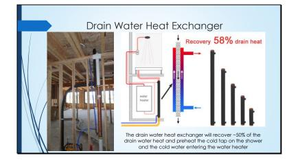
The drain water heat exchanger is another way we can temper the water before it enters the hot water heater. It only works when you are draining and drawing at the same time (showers). But the cold water at the shower mixing valve is warmer, so you don't use as much hot water. The water entering the tank is also much warmer.
