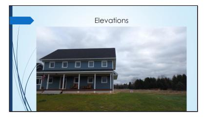
South side of the house has 24" overhangs on the 2<sup>nd</sup> floor and 36" overhang on the 1<sup>st</sup> floor for summer shading.
