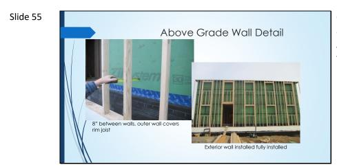
Outer wall covers the rim joist, and sits on the foundation wall. All of the RO for the windows are framed in the outer wall.
