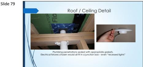
There are 2 penetrations in the 2<sup>nd</sup> floor ceiling – 1 plumbing stack sealed with a rubber gasket and a coax cable to an HD antenna in the attic – also sealed with a rubber gasket. All of our lighting is surface mounted – and the "recessed lights" we used fit in standard junction boxes.
