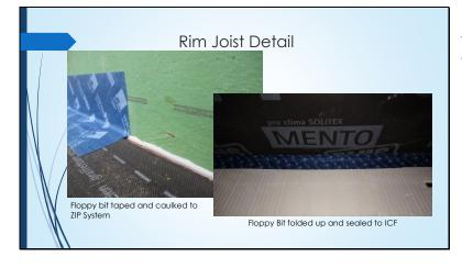
Floppy bit sealed to above grade wall air barrier and to foundation wall air barrier.
