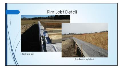
1<sup>st</sup> floor deck set on top of floppy bit. Rim board installed
