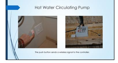
The circ pump was installed because of the distance between the master bedroom and location of the water tank. It also makes the water heater that much more efficient. When you drain the cold water from a the faucet – the water in the tank is replaced with street temperature water (about 40-50 degrees). When you turn on the circ pump, the water in the loop is roughly 70 degrees. You water heater doesn't have to work as hard.
