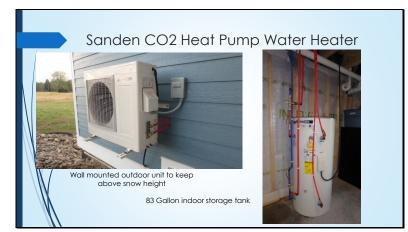
The water heater is a split heat pump. A standard heat pump water heater would double the heat load for the house – as the byproduct of the heat pump water heater is air conditioning.
