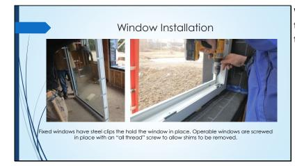
We planned to ½" gap to allow us to adequately foam the window to the RO.
