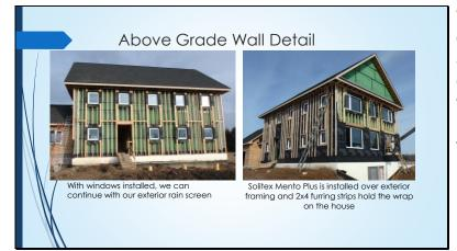
With the windows installed, we can finish our above grade wall assembly. We covered the exterior framing with our weather resistant barrier, and installed 2x4 furring strips over that to hold it in place
