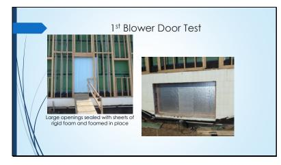
1<sup>st</sup> Blower Door prep – sealed all openings with rigid foam prior to test
