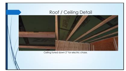
We furred down the 2<sup>nd</sup> floor ceiling 2" to allow an electrical chase and overhead lighting
