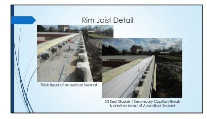
Belt and suspenders – acoustical sealant, sill plate gasket, acoustical sealant.
