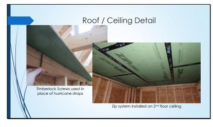
Hurricane straps would be problematic with an OSB ceiling – we used the Timberlock screws. Much Faster and Easier! After the roof was on, we sheeted the ceiling with Zip and tape all seams.
