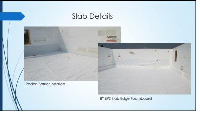
Radon Barrier laid flat
