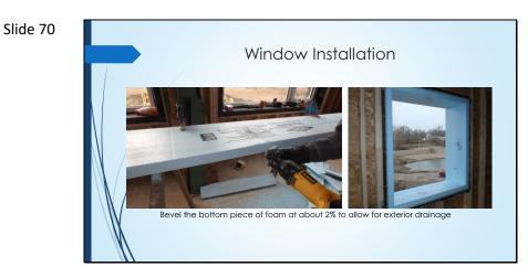
We tapered the bottom foam to allow for drainage.
