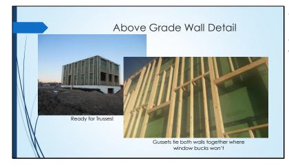
8" space between walls – to be insulated with dense packed cellulose. Gussets tie the walls together.
