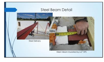
Steel Beam pocket insulated with rigid foam – R-25.7 to the outside of the steel
