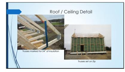
Trusses sit on the zip system gusset. We have over 24" at the outside edge of the outside wall to ensure our continuous thermal envelope.
