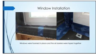
Then we sealed the window to the weather resistant barrier and the weather resistant barrier to the flashing tape we installed in step 1.
