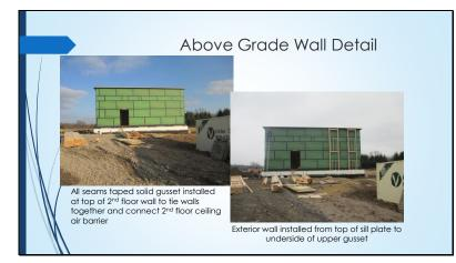
Gusset installed at the top of the 2<sup>nd</sup> floor wall to tie the inner and outer walls together. Outer Wall built
